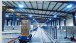
■ Intelligent three-dimensional warehouse
